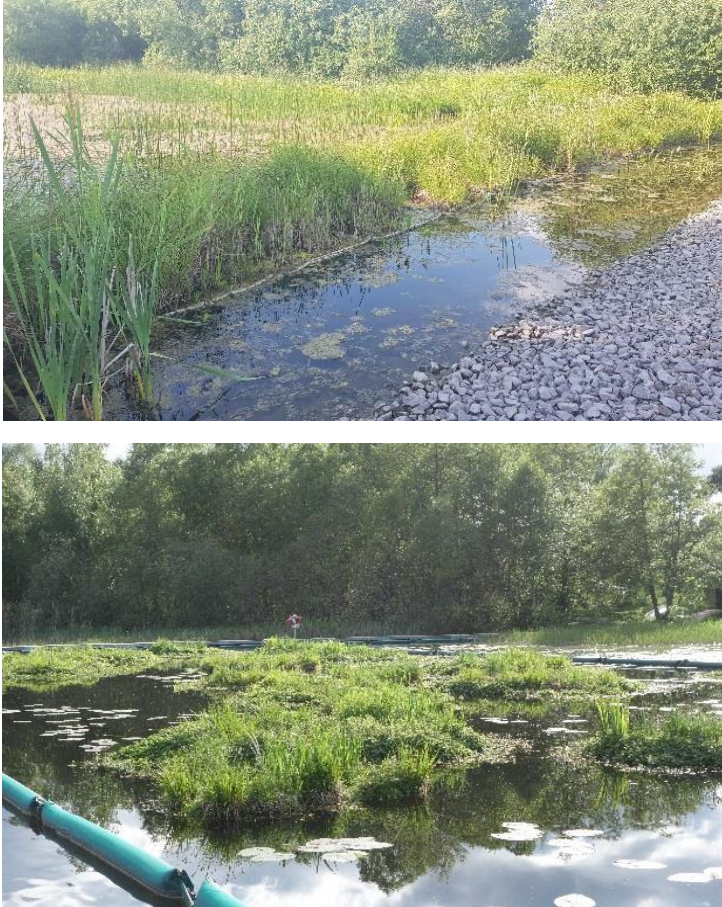
Figure 5. Floating treatment wetlands in Norra Sörentorp stormwater pond, installed 2011 (top), and lake Rönningesjön, installed 2013 (bottom).
