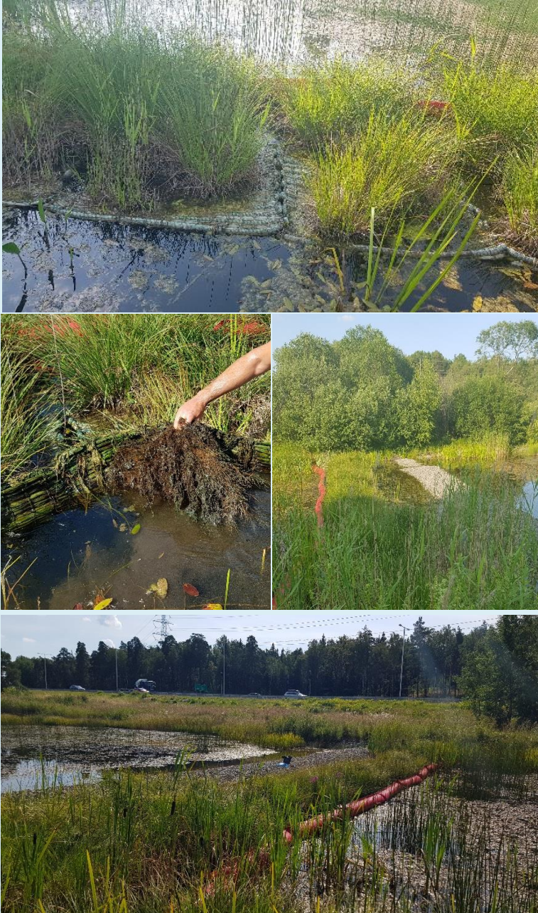
The long and narrow FTW is placed across the Norra Sörentorp stormwater pond close to E4 highway in northern Stockholm. Some gaps in the vegetation expose the plastic mat of the raft. Dense root mats have formed beneath the raft.
